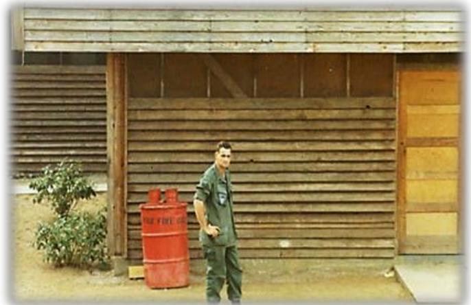
458 th HQ Bldg/Supply Room
